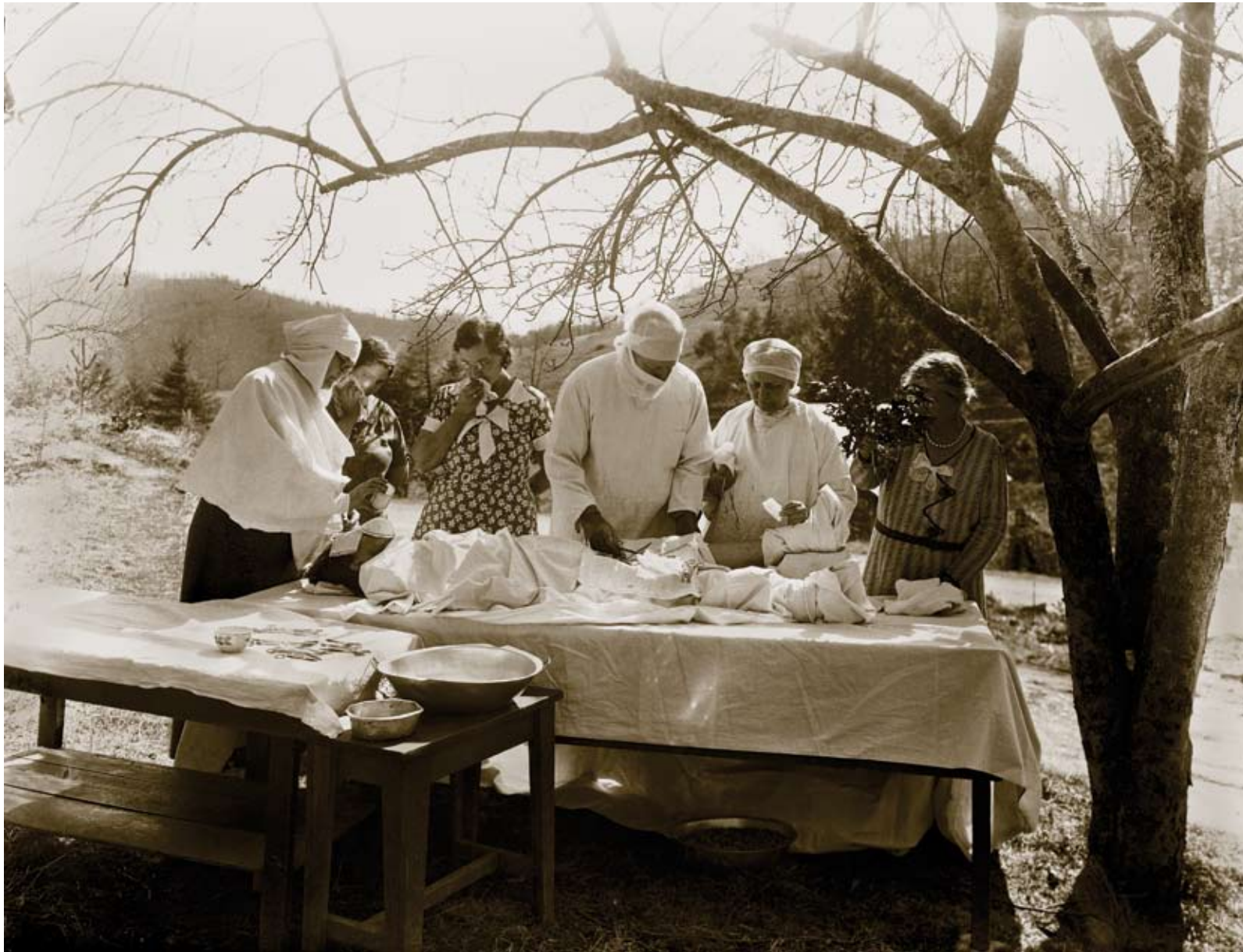
Surgery in Avery County about 1920. In early 20th-century North Carolina, there were few hospitals and poor roads, so rural doctors were often forced to treat patients under primitive conditions. Photo by Bayard Wootten, courtesy of the North Carolina Collection, University of North Carolina at Chapel Hill.
